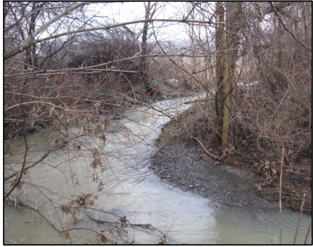
12' CONC. ELLIPTICAL CULVERT
