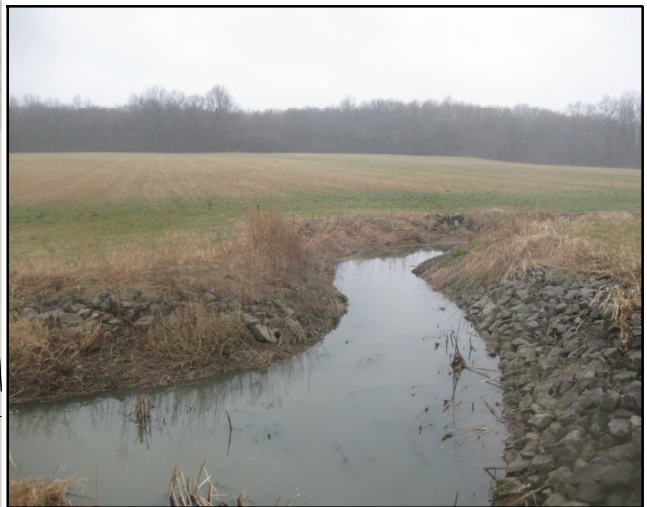
5'x14' CONC. BOX CULVERT
